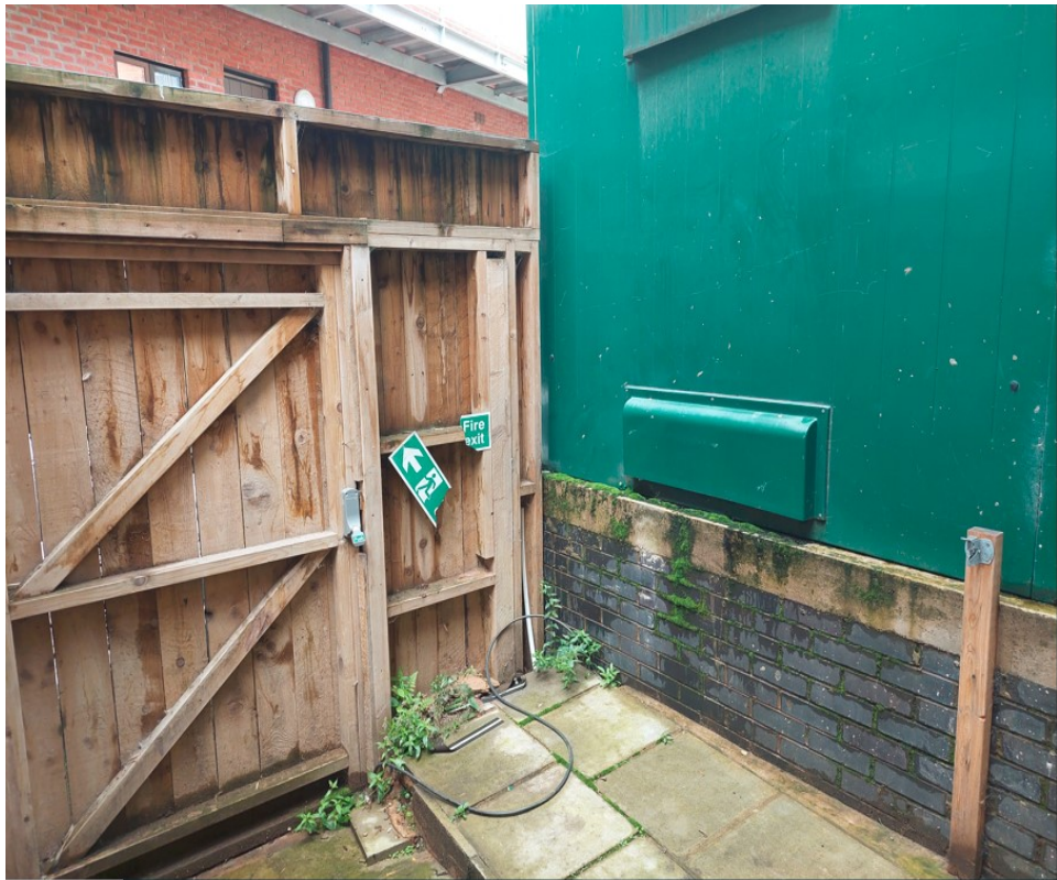
- Fire exit in the rear yard of 11 Castle Foregate (current premises) -
