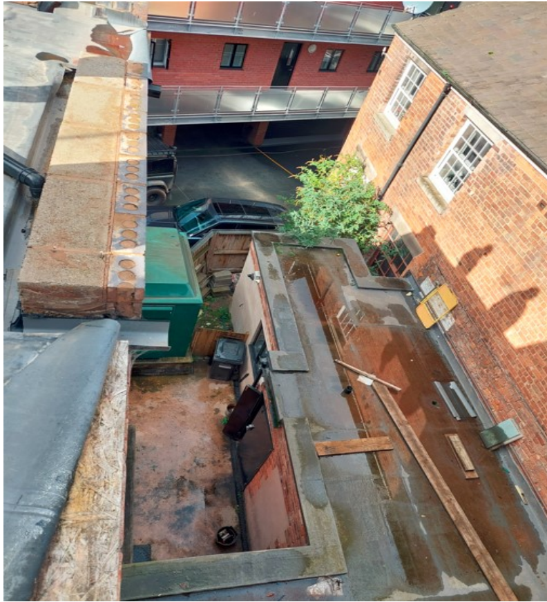
- Aerial view of the rear yard, 11 Castle Foregate (current premises) -
